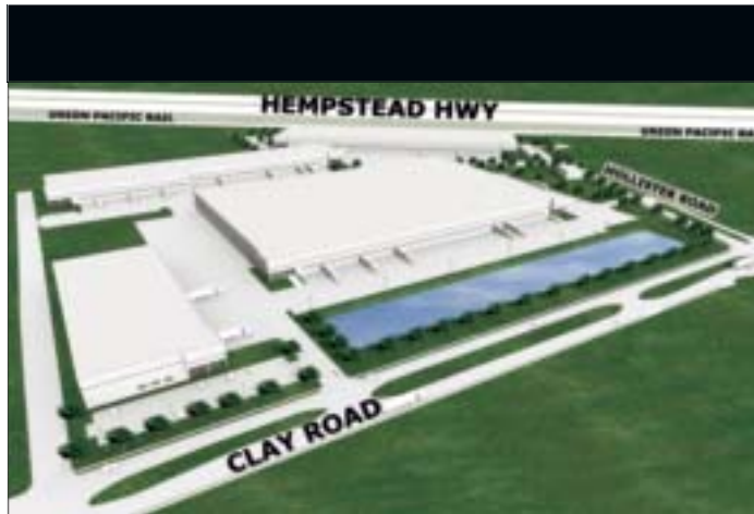
The Houston office of Cadence McShane has been selected by Weingarten Realty to construct two new industrial facilities totaling nearly 300,000 square feet at the developer's ClayPoint Distribution Park located in northwest Houston, Texas that will be completed in Third Quarter 2008.
