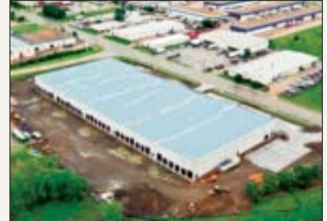
NORTHFIELD 800 – GRAPEVINE, TX
