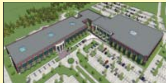
Cadence McShane has been selected to construct the new 150,000 square foot, two-story office headquarters for Torchmark Corporation located on an 18-acre site in McKinney, Texas with completion scheduled for November 2007.
