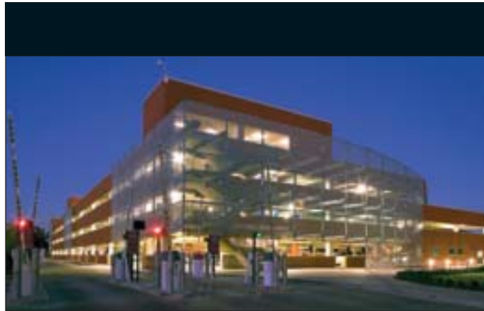
Two 1,000-car, 340,000 square foot parking garages were recently completed by the joint venture between Diggs Construction, LLC and Cadence McShane on the campus of Texas Southern University in Houston, Texas.
