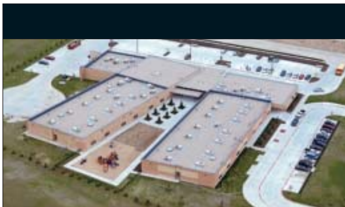
On behalf of the Carrollton-Farmers Branch Independent School District, Cadence McShane recently completed the new 47,500 square foot Kelly Pre-Kindergarten Center in Carrollton, Texas four weeks in advance of the agreed upon delivery date.
